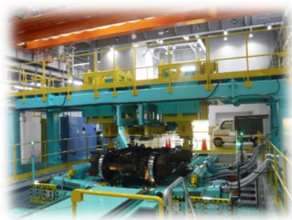
Mechanical equipment for Railway Company
