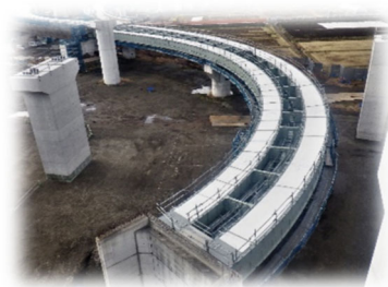
Yokohama Loop Line H-ramp No.1 bridge
