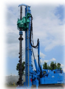
Pile driving rig
