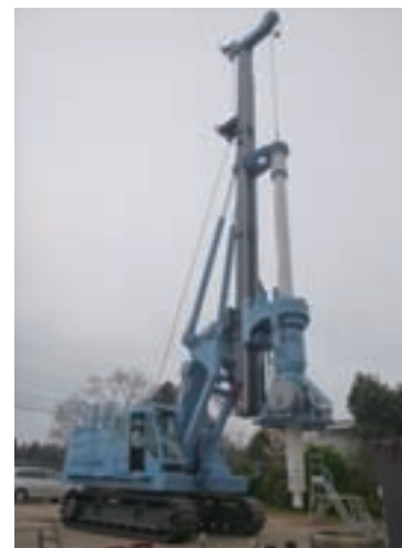
Pile driving rig
