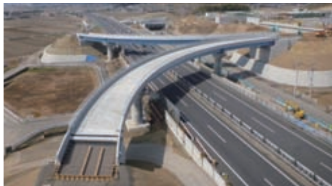
Kita-Kanto Expressway Ota Parking Area Ramp Bridge
