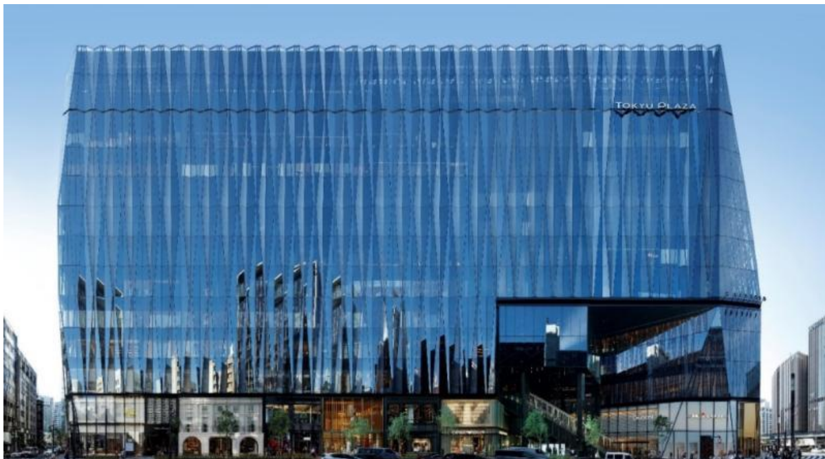
建物外観 © Koji Fujii / Nacasa&Partners Inc.
